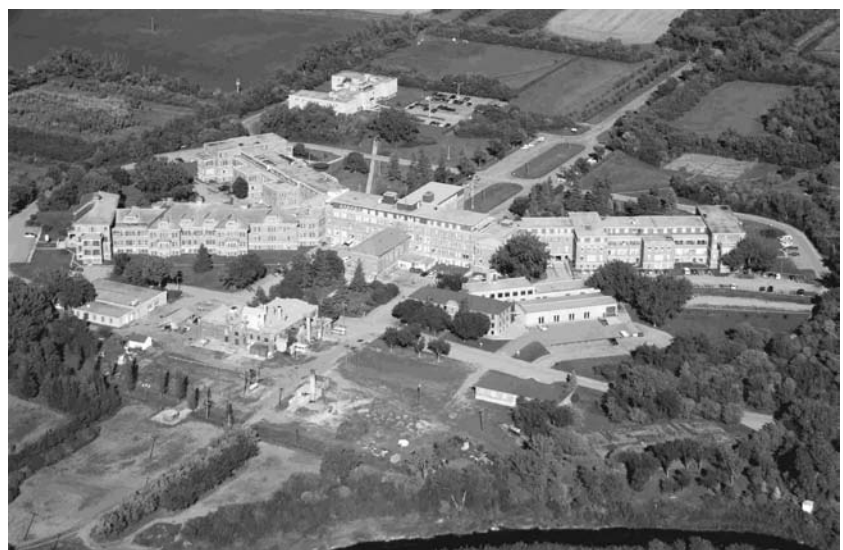
The mental hospital in Weyburn may be converted into sales offices, showrooms and a shipping distribution centre for Chinese goods.
